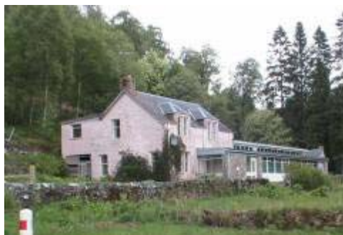
Fig. 3 : Original building and extensions
